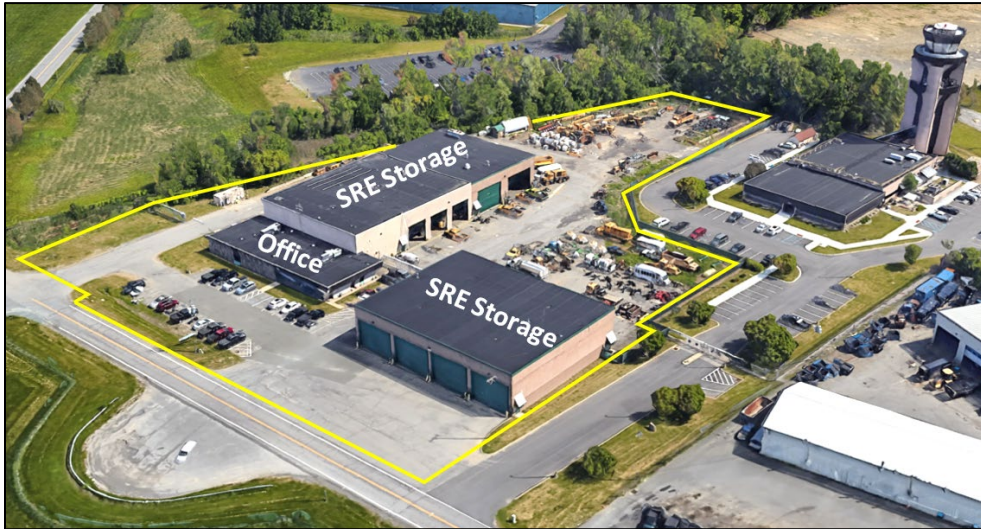
Figure 4-13 – SRE & Maintenance Buildings
