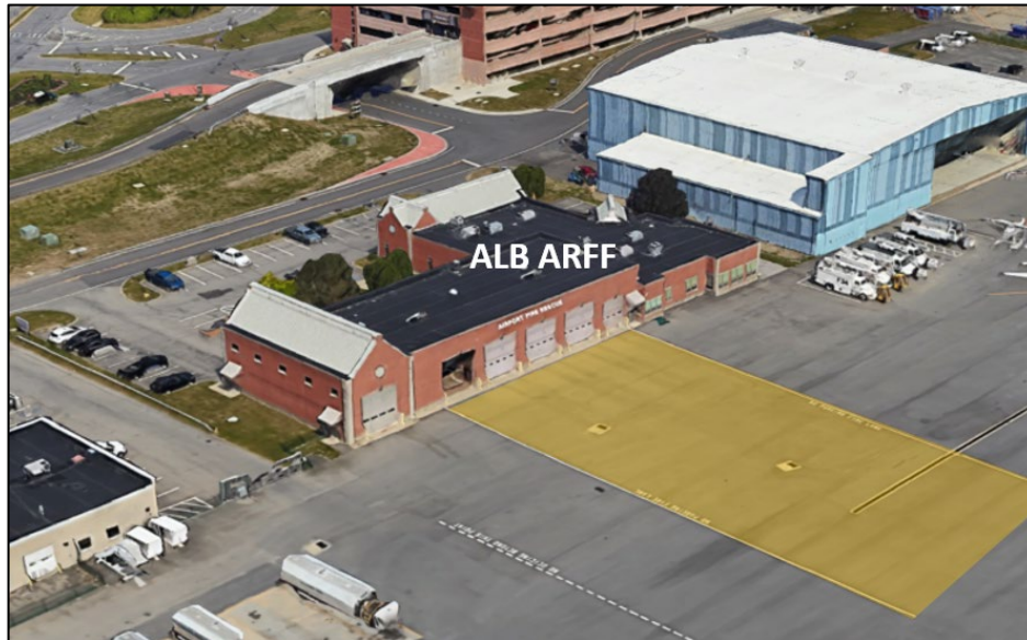
Figure 4-14 – Existing ARFF Station
